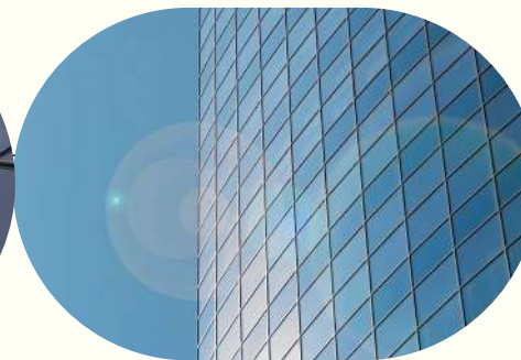
Utilities, associations, and consortium
